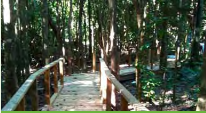
Cinnamon accessible trail under construction.
